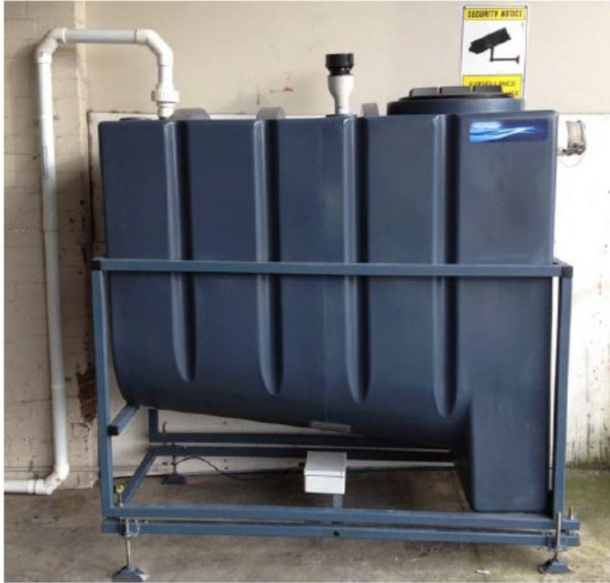
Figure 4 Pulpmaster Bio-digester holding tank.
